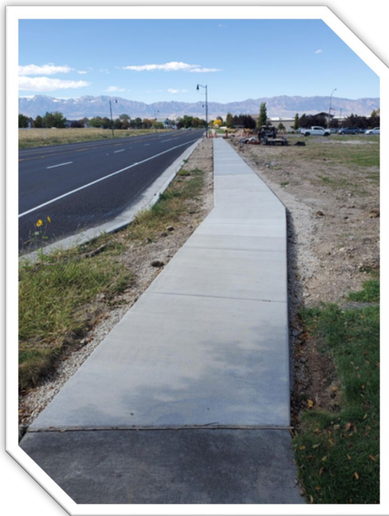
New Sidewalk along 2000 North
