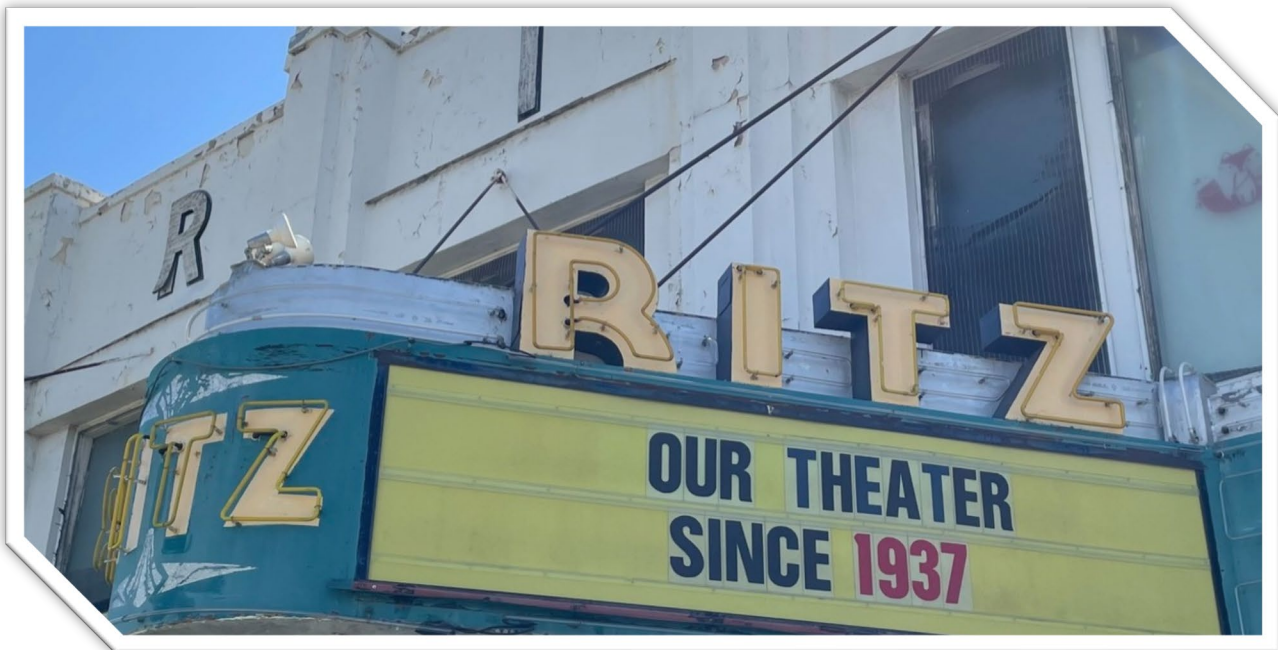
Ritz Theater Renovation
