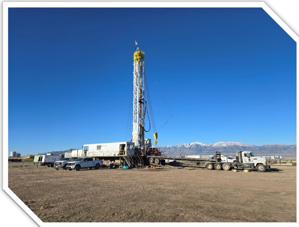
Drilling the New Rogers Street Production Well March 2026
