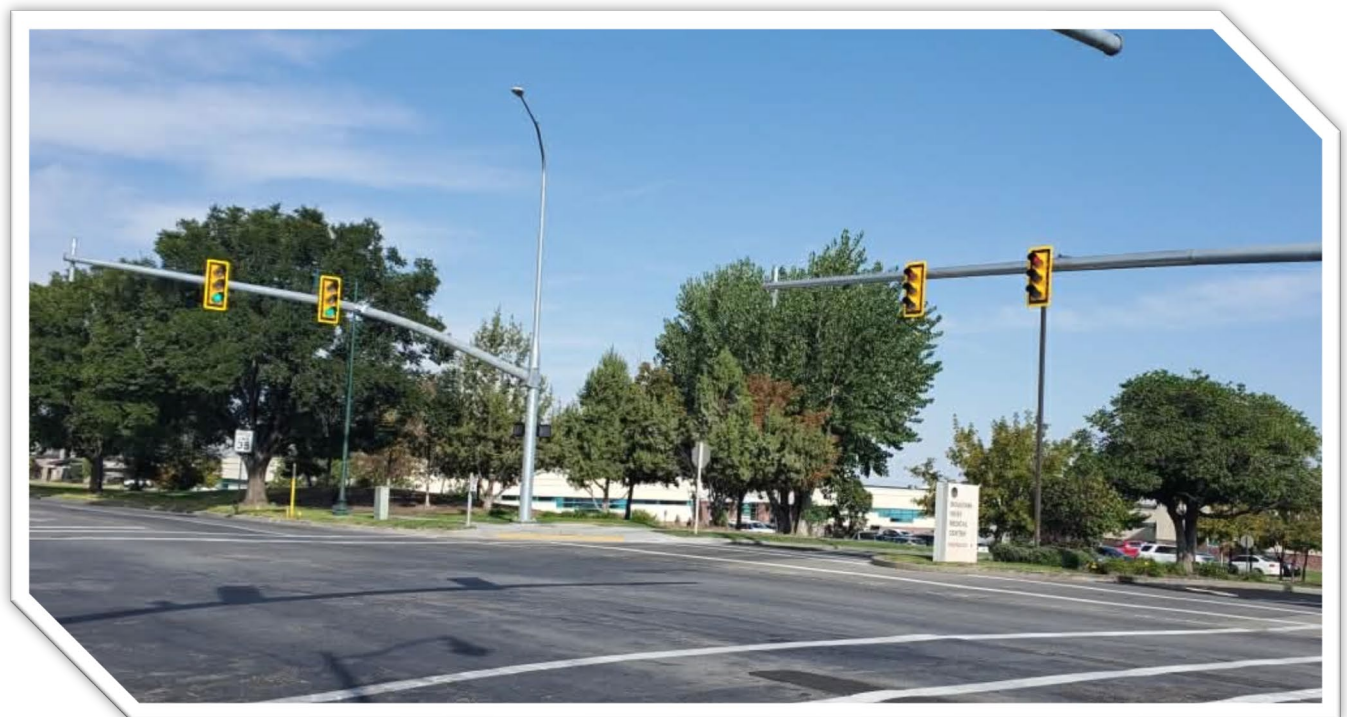
As our City continues to grow, so does the importance of assessing and improving traffic safety. A new traffic signal was installed at Aaron Drive and 2000 North in September 2025.
