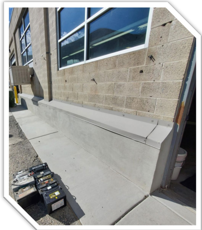
Fleet Building - New concrete wall and apron
