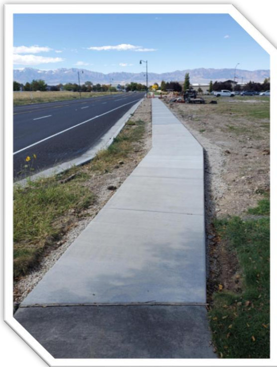
New Sidewalk along 2000 North
