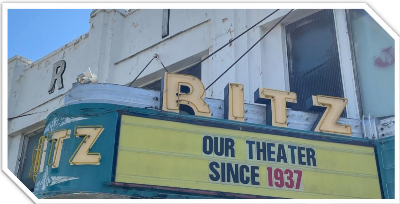
Ritz Theater Renovation
