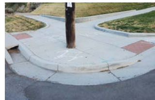
Directional curb ramps
