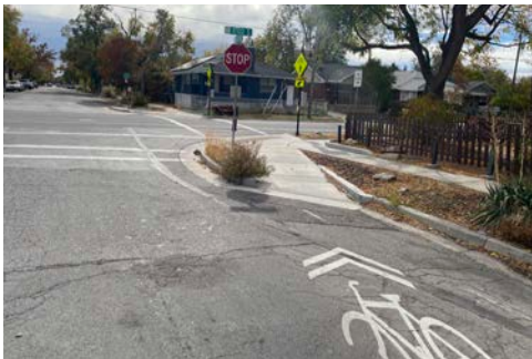
Bike Ramp Bulbout to Crossing - SLC, UT
