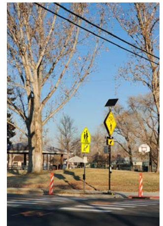
High-visibility crossing with flashing beacon
