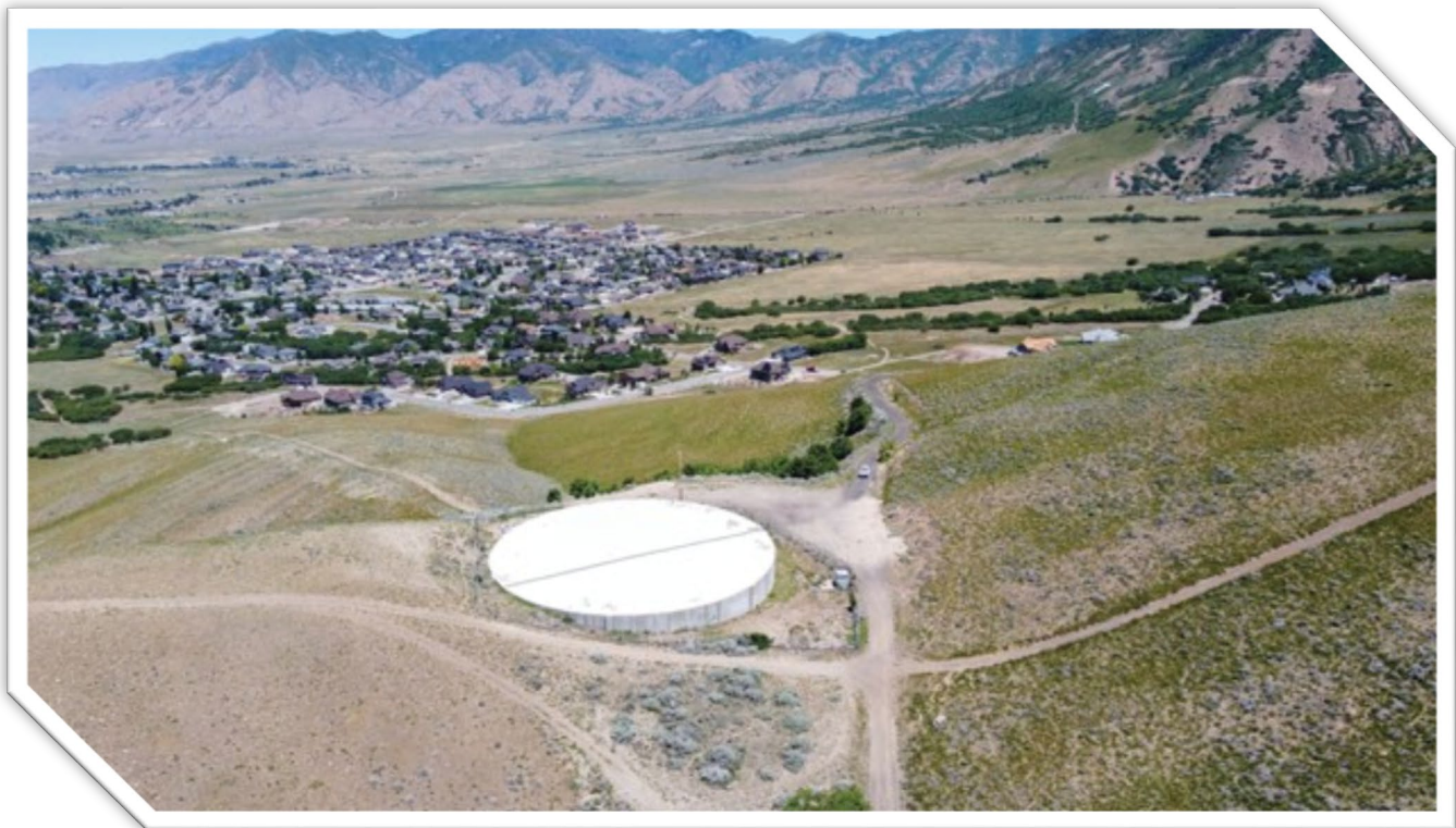
Water tank above Tooele City
